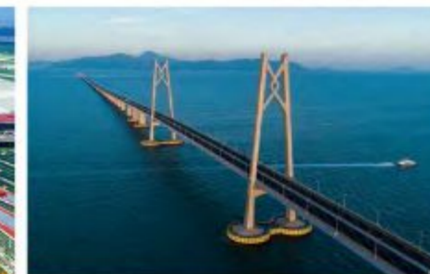
Hong Kong-Zhuhai-Macao Bridge
