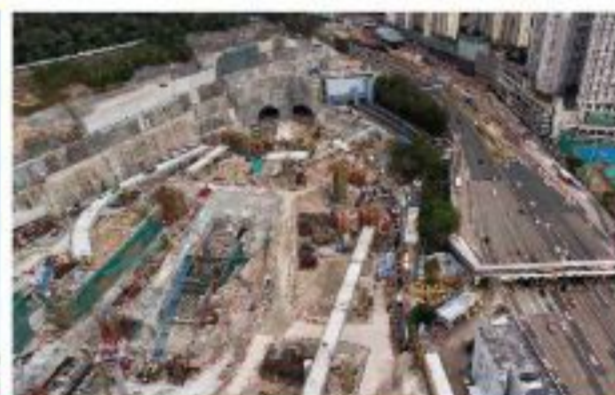
Lam Tin Tunnel project
