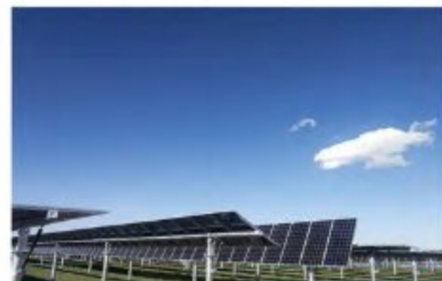
Qinghai 10 Million Watt PV Project
