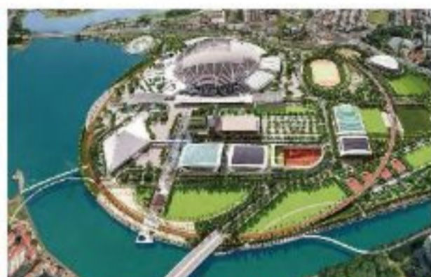
Kallang Football Facility
